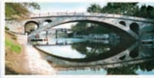
▲ **A.D. 600** Chinese Emperor Yang Ti oversaw the construction of the An Ji Bridge. It was the first of its kind, called an open-spandrel arched bridge.
